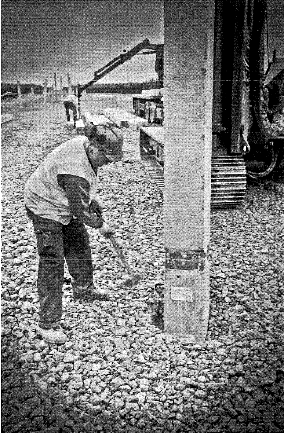
Figure 9: Installation of the locking pins
