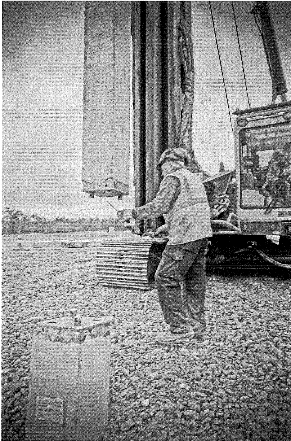
Figure 8: Joining pile sections
